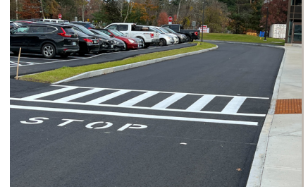
Above: Site work painting and striping.
