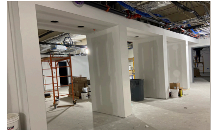
Above: 2nd Floor Teams Area entrance from corridor.
